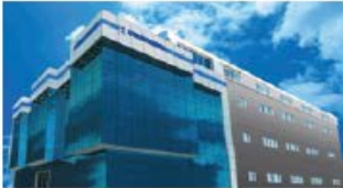
Fabrika / Factory - İstanbul Atatürk Cad. Çağatay Sokak No:3 Sarıgazi Sancaktepe / İstanbul / TURKEY 34785 Tel. / Phone : +90 216 499 14 64 (Pbx) Faks / Fax : +90 216 499 66 19
